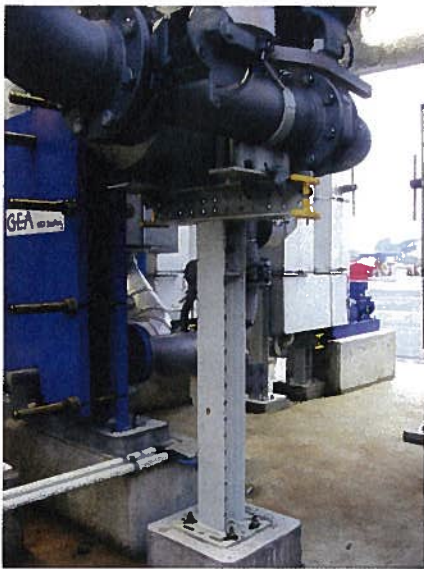
Use of the carrier 100 and height-adjustable seat for the high load range
